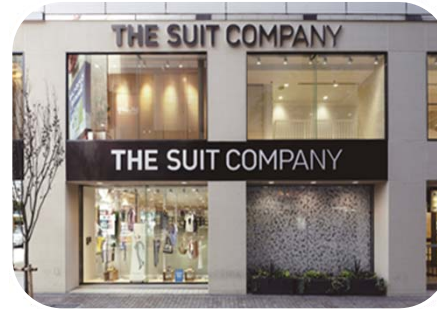
TSC in station side Building
